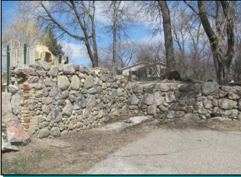
Retaining wall deterioration at Neighborhood 8
