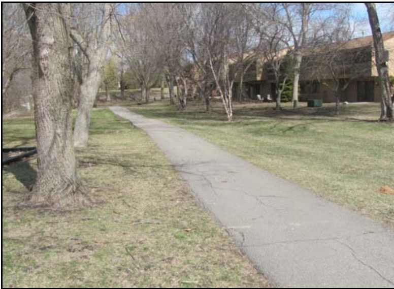
Cracks in walking path at Neighborhood 1
