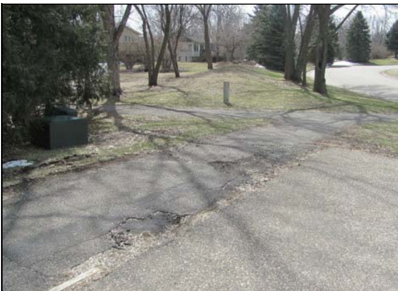
Walking path deterioration at Neighborhood 8
