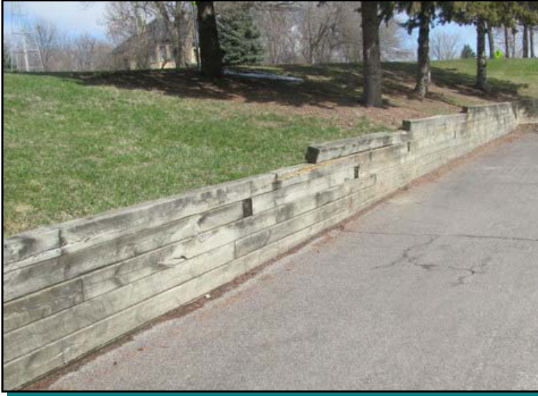
Wood retaining wall deterioration at Neighborhood 1
