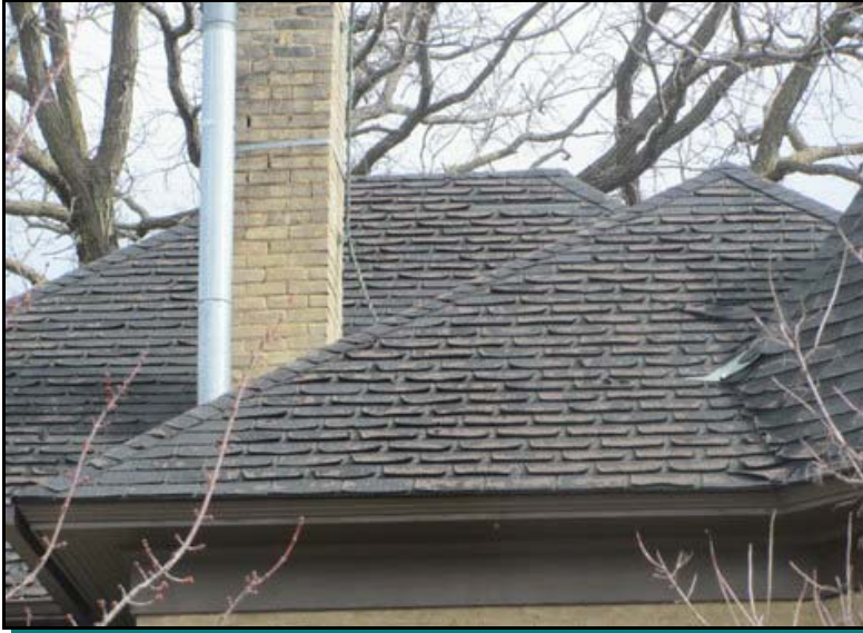
Shingles in poor condition
