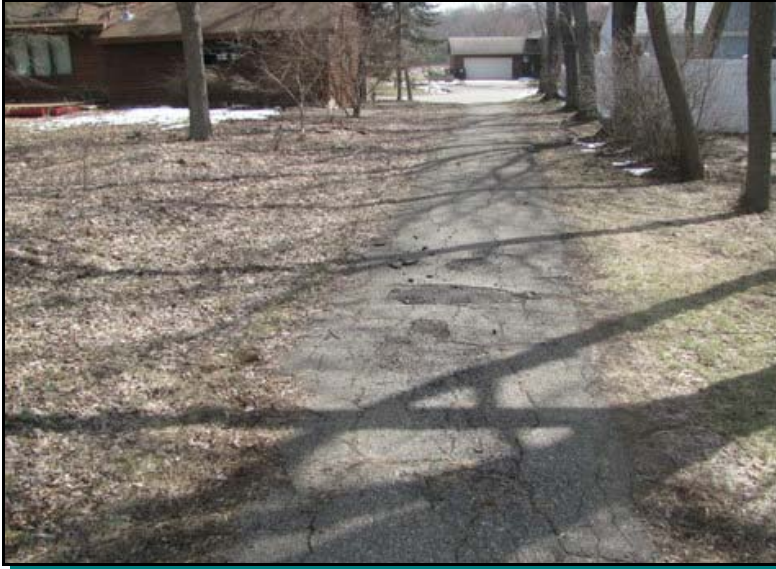
Walking path deterioration at Neighborhood 8
