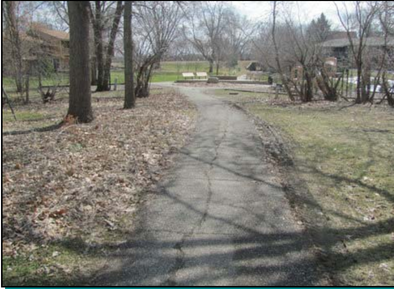
Cracks in walking path at Neighborhood 1
