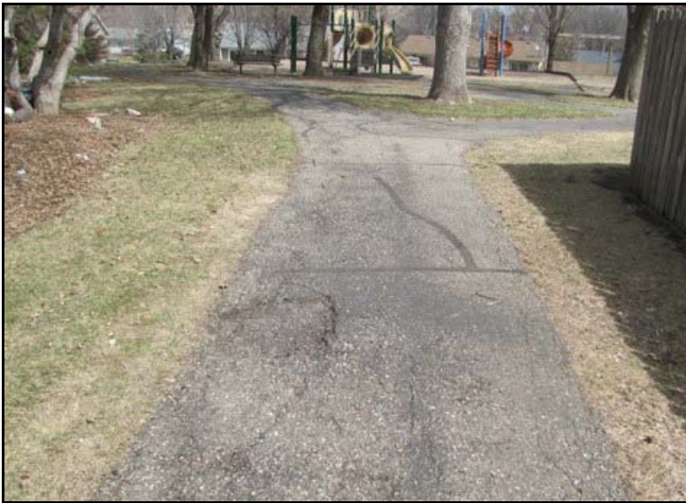
Walking path deterioration at Neighborhood 9
