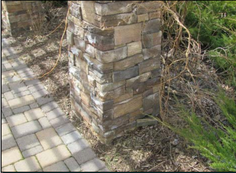
Delaminated masonry - fund repairs through the operating budget
