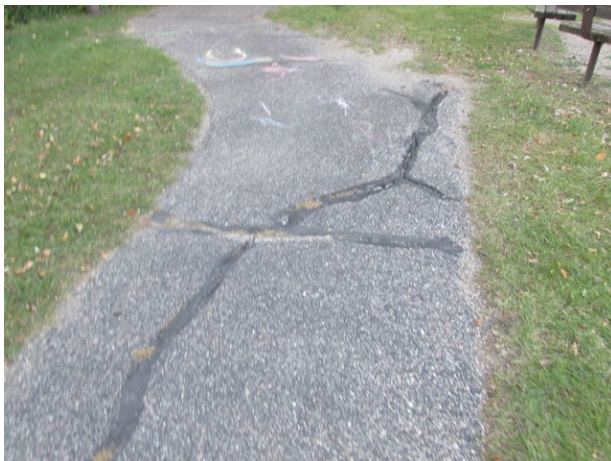
Walking path crack repairs at Neighborhood 5
