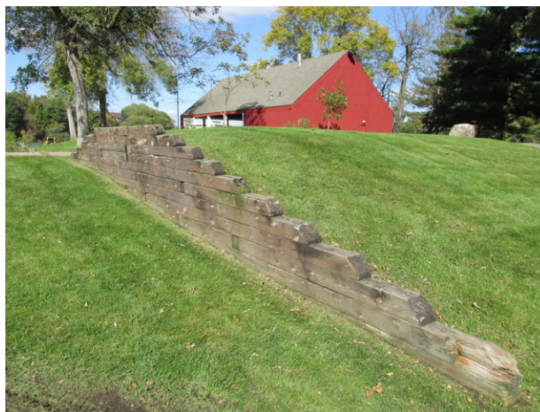
Leaning timber retaining wall near pavilion
