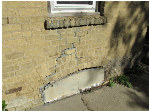
Masonry deterioration and typical step cracks at Eitel House
