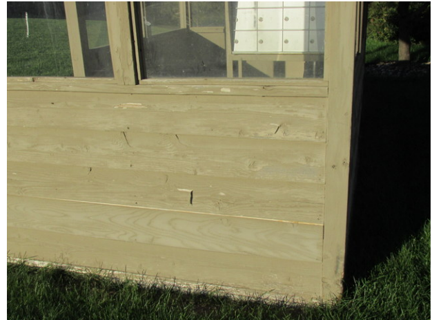
Paint finish deterioration at mailbox pavilion at Neighborhood 10
