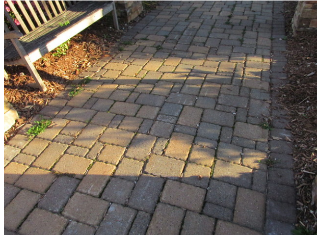
Minor settlement at brick pavers
