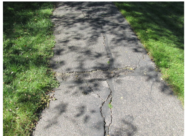
Asphalt pavement failure at Neighborhood 6
