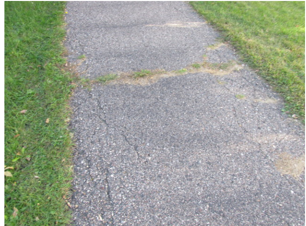
Pavement deterioration at Neighborhood 7
