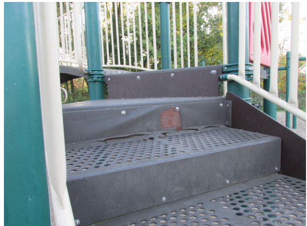
Coating deterioration at playground stairs at Neighborhood 11
