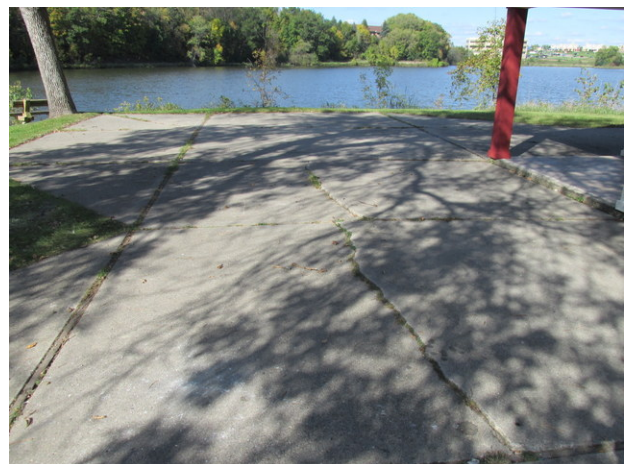
Concrete deterioration at pavilion
