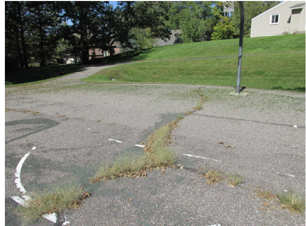
Surface cracks and deteriorated pavement
